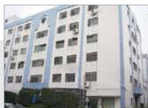
MEAN WELL GUANGZHOU TIANHE R&D CENTER
